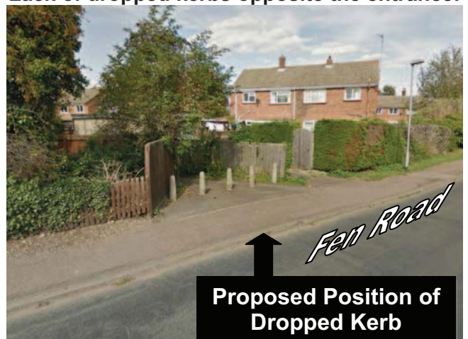
Photo 2 – Lack of dropped kerbs opposite the entrance:
